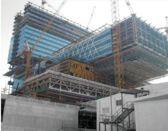
Flat roof, Terraces
