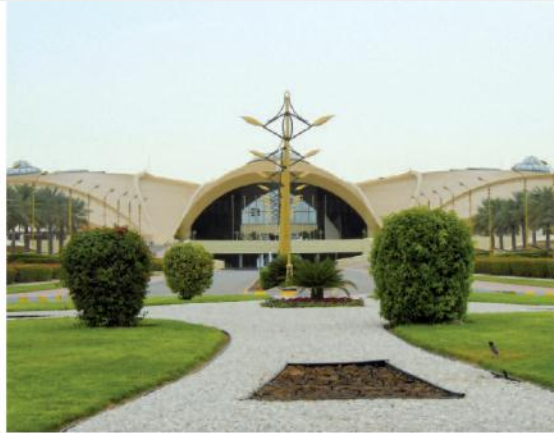
Roof with metal covering
